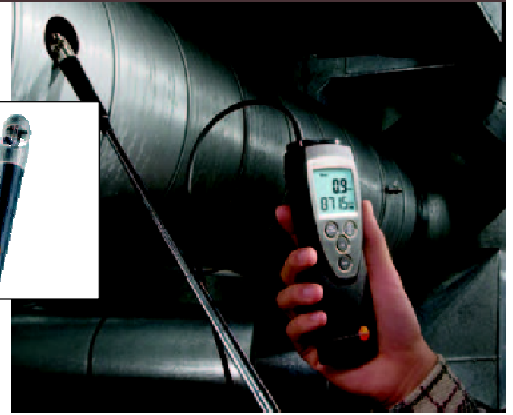
Monitoring air velocity in air conditioning ducts
